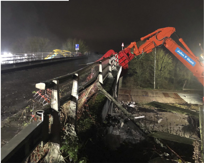
Images of the old Generals Lane bridge over the railway line and A12 slip road being demolished
